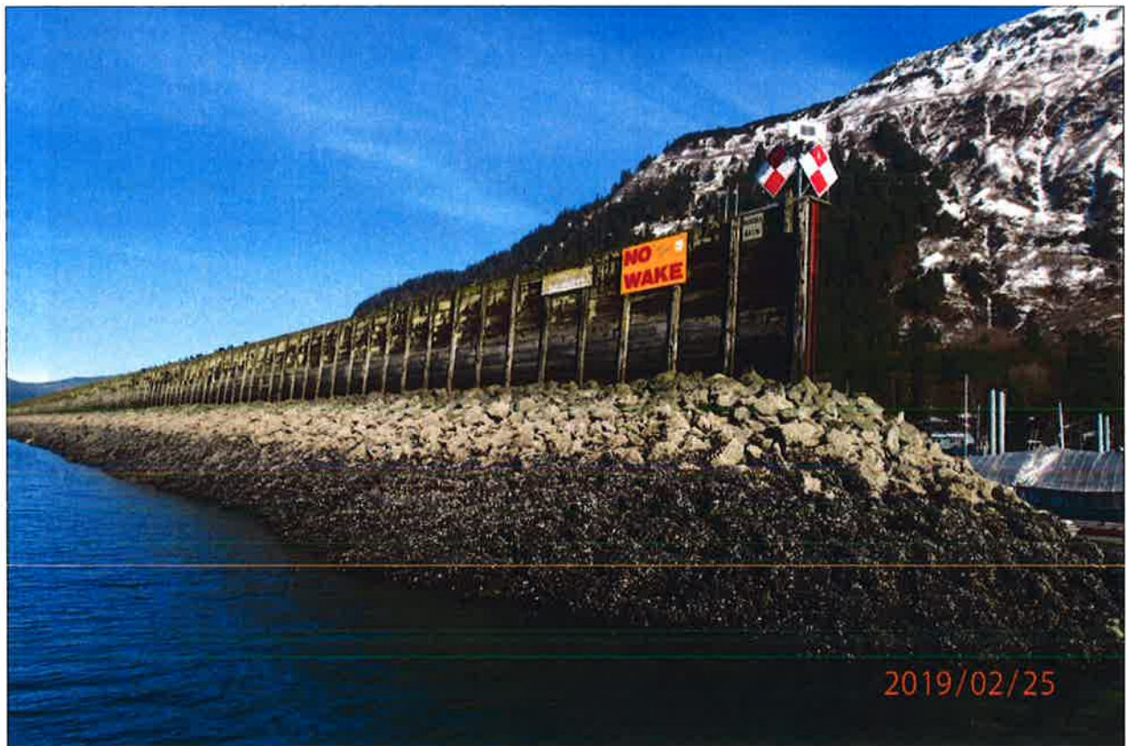
Figure 5. Composite wave barrier at Aurora Harbor, Juneau (USACE 2019).
