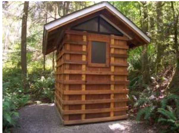
Composting toilet installed along a trail
