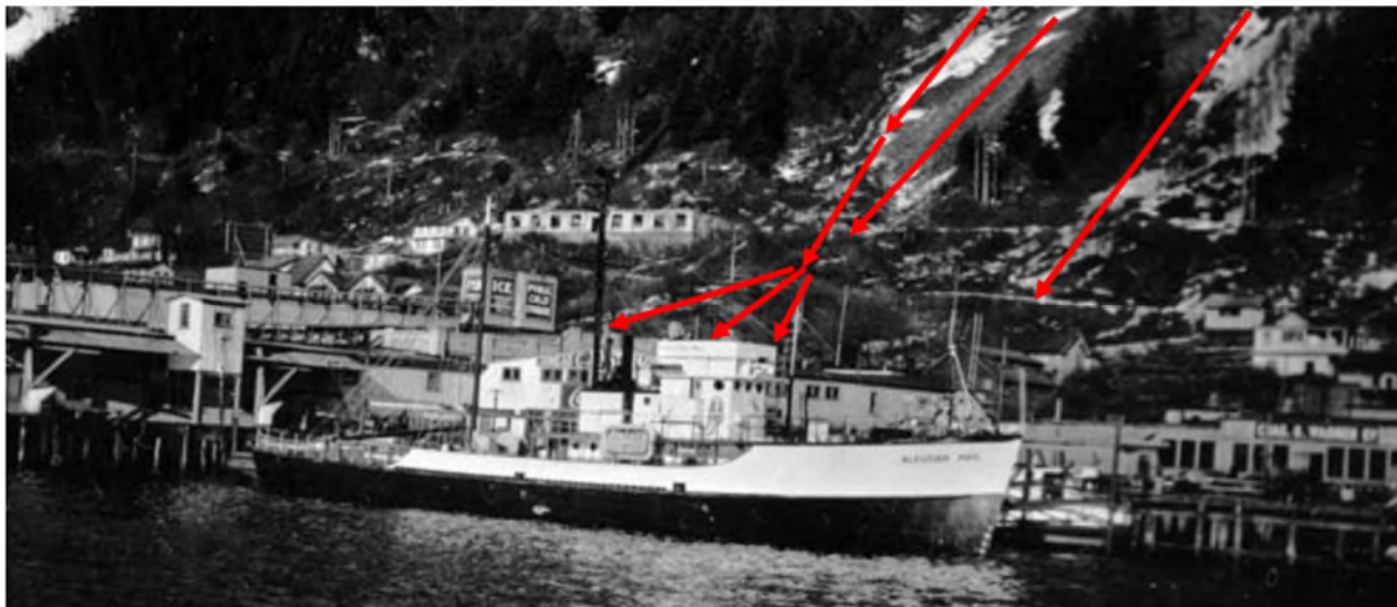
Figure 6: Two apparent debris paths from November 22, 1936, landslide (red arrows, see also Figure 1a, 1b attached). Structure at center-left was the Juneau Cold Storage Company building, later replaced. Debris ran up against the S. Franklin St. side of Juneau Cold Storage, moved the Madsen Building downslope, destroyed several buildings, and killed 15 people. (Photo credit: Alaska State Library – Historical Collections, ASL-P134-312-4 , date uncertain, cropped to fit. ASL 2022d.)
