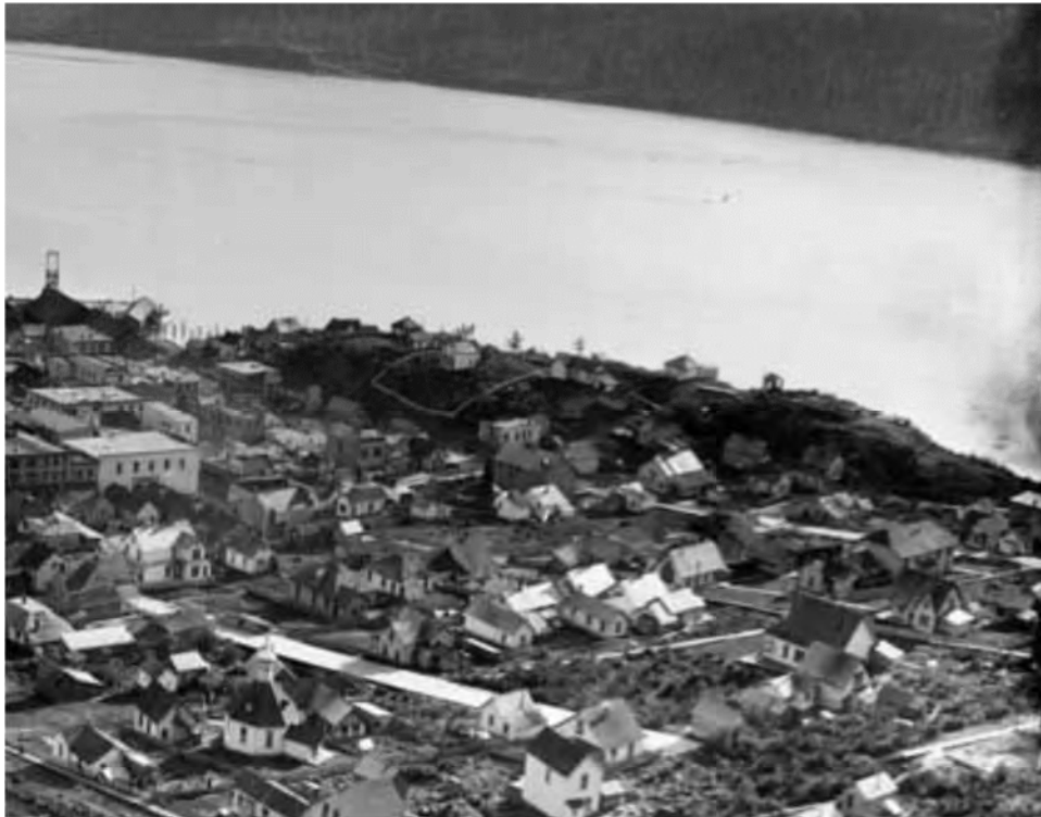
Figure 1: Looking south towards Telephone Hill and Gastineau Channel from Mt. Maria, circa 1896, early in the development of Juneau, when structures along the toe of slope at Willoughby Avenue were supported on wharfs, and before fill began to be placed along the shoreline to extend the useable land area. (Photo credit: Excerpted from Alaska State Library – Historical Collections, ASL-P87-0753 , Winter & Pond, ca. 1896.)
