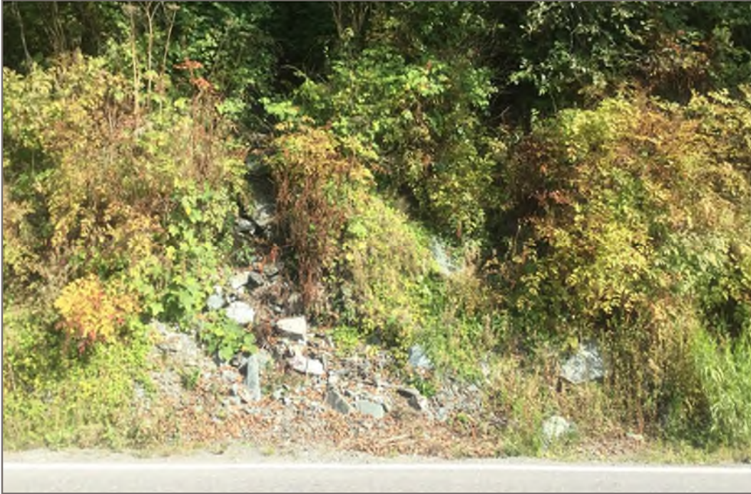
Photo 13: Looking northeast across Thane Road. This is an example of a debris flow that has essentially stopped at the upslope edge of Thane Road. Material transited through the same gully pictured in Photos 9 to 12. (Date of Photo: September 9, 2019; The photo location is shown on Figure 2). , 2019; The photo location is shown on Figures 1.4 and 1.5).
