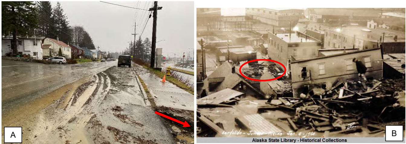
Figure 13: These photos are of Moderate terrain. Figure 13A is looking southeast along Glacier Avenue on December 4, 2020, where Ross Way enters. Ross Way carried debris and water from Behrends Avenue to Glacier Avenue. Debris can also run southeast on Behrends Avenue. Note the apparently eroded and failed section of the sidewalk (at red arrow) where a section of concrete slab was missing. Figure 13B is looking downslope towards South Franklin Street (formerly Front Street) on January 2, 1920, after a major landslide from upslope of Gastineau Avenue. The red circle shows possible landslide debris across the street. (Photo credits: Figure 13A: CBJ December 4, 2020. Figure 13B: Alaska State Library – Historical Collections, ASL-P109-42 , Katherine Shaw 1920. ASL 2022b.)
