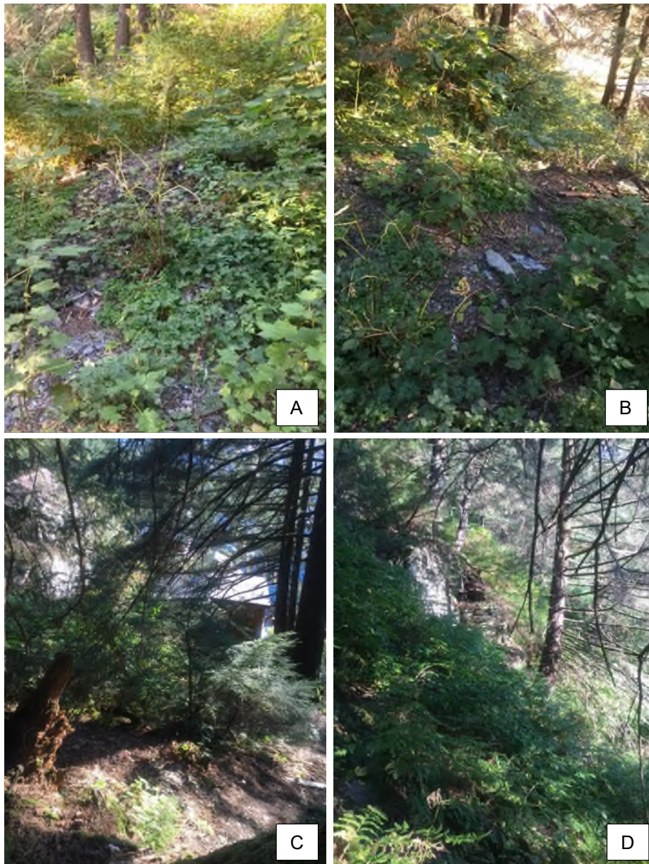
Figure 9: Active debris slide paths above Nelson Street are shown in Figures 9A and 9B; rock bluffs and broken or damaged trees above Nelson Street are shown in Figures 9C and 9D.
