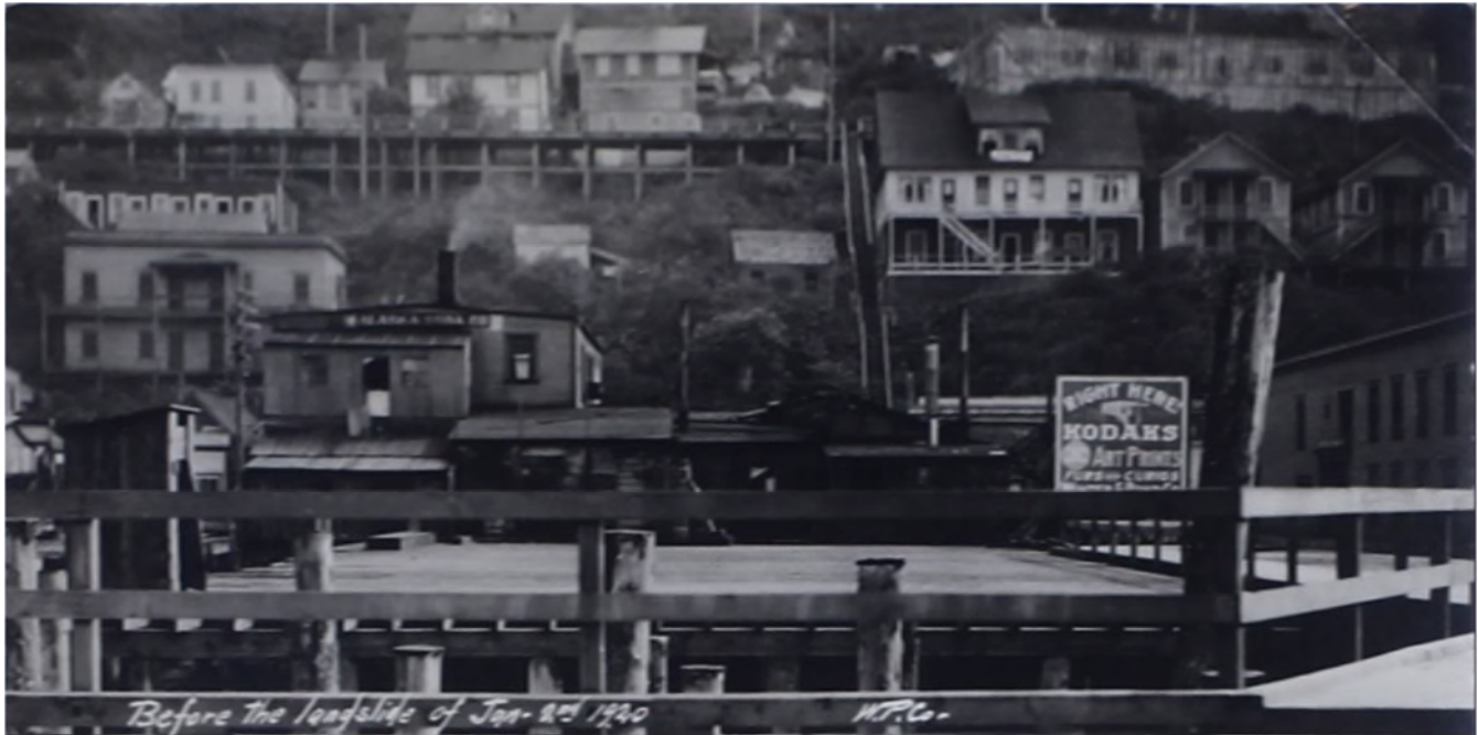
Figure 4: This “before” photo is from after 1914 but before 1920, and possibly from the summer of 1919. The stairway at center-right is Bulger Way. The pier-like structure is Gastineau Avenue. Decker Way (a stairway) is located just beyond the left edge of the photo. Note the numerous structures between Decker Way and Bulger Way before the landslide. Just up and left of the smoking-chimney building is the tenement building that tipped and rotated clockwise during the landslide (see Figure 5). Top right is the former Alaska Juneau Gold Mining Company (AJGMC) office building. (Photo credit: Alaska State Library – Historical Collections, PCA0154-295, Snow Family Photograph Collection. ASL 2022b.)
