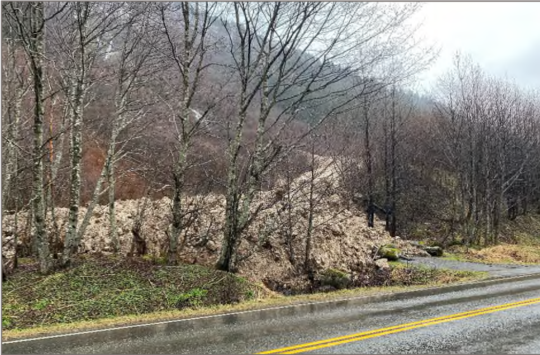
Photo 23: Looking upslope (northeast) from Thane Road into the Snowslide Creek (T011) avalanche path (Photo Credit: CBJ Dec 4, 2020. The photo location is shown on Figures 1.4 and 1.5). Wet avalanche flow was diverted by the earthfill diversion berm toward the northern boundary of the Severe (red) hazard zone.
