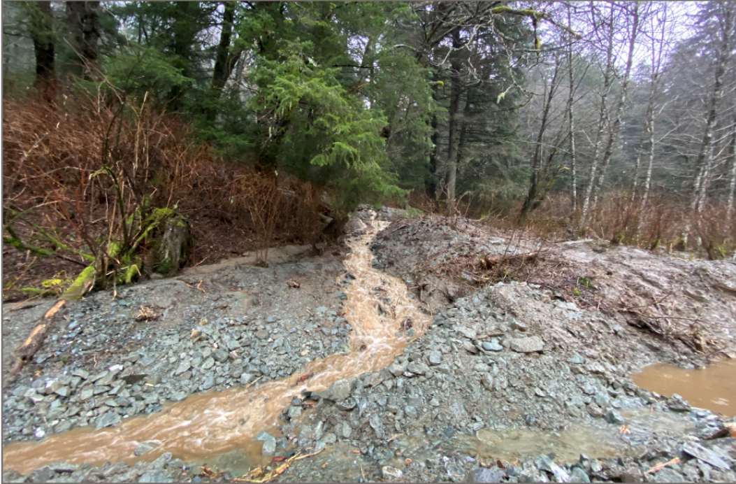
Photo 19: Looking southeast and upslope at debris flow material depositing on Glacier Highway above the AWARE shelter (Photo Credit: CBJ Dec 4, 2020; The photo location is shown on Figures 1.4 and 1.5).
