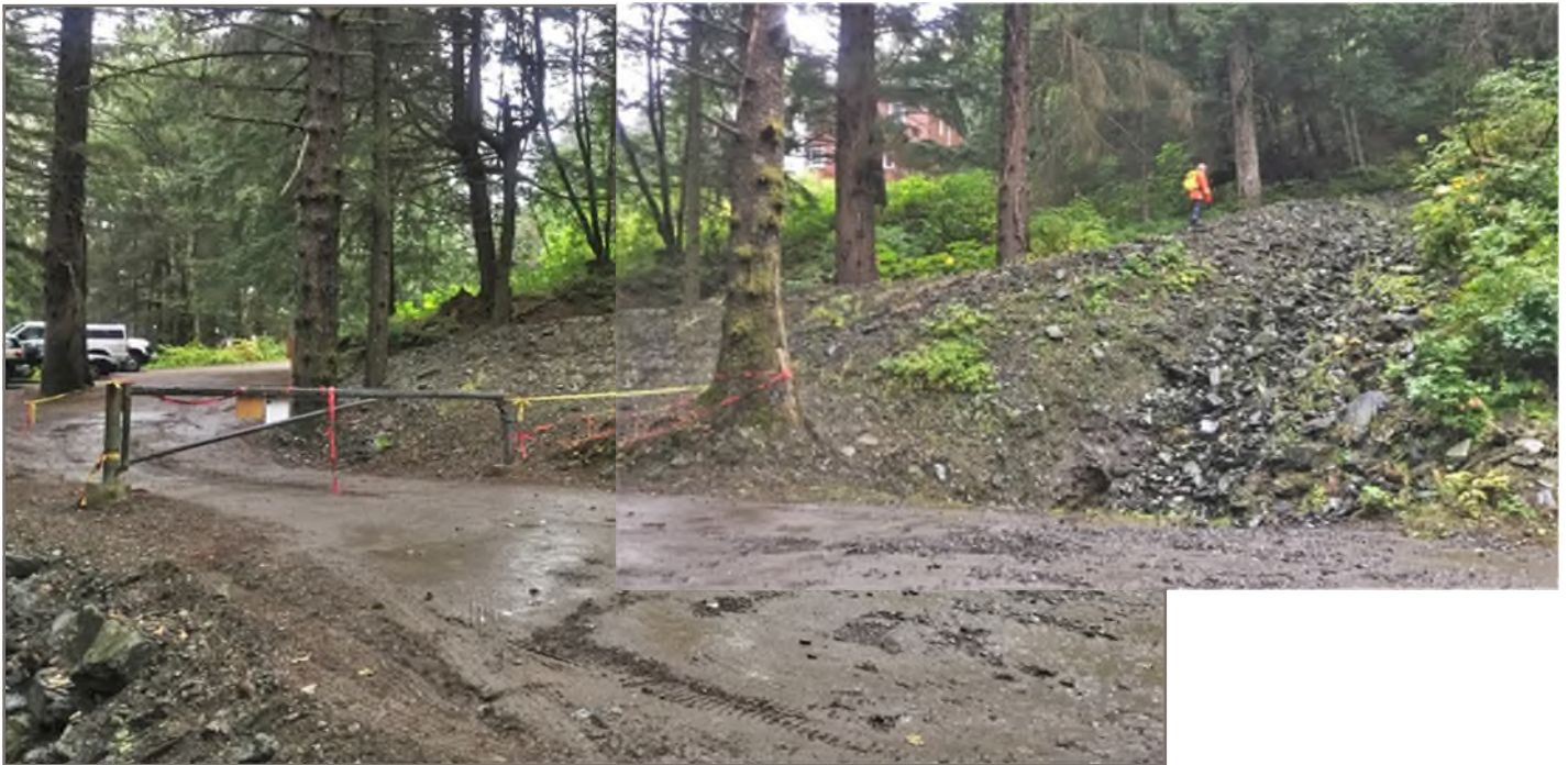
Photo 16: Looking west and across slope at debris flow material deposited near the end of Evergreen Avenue. A recent debris flow has partially buried some of the tree trunks. (Date of Photo: September 11, 2019; The photo location is shown on Figures 1.4 and 1.5).
