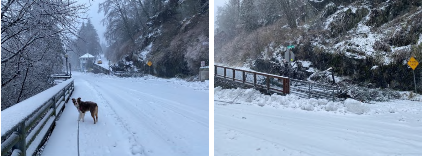
Figure 3: Typical debris slide deposit at the fork between Dixon Street and Calhoun Avenue. In the left-hand photo, note the fork in the road at center-right, and the northwest end of the retaining wall at the right edge of the photo. The downslope edge of Calhoun at the railing is supported by another retaining wall. In the right-hand photo, note the presence of a steep cutslope into apparent weathered bedrock, with a thin veneer of colluvium. The debris from this landslide event extends an estimated 40 feet northwest of the end of the metal railing. The distance along the toe of slope along Dixon/Calhoun is about 110 feet between the northwest edge of the debris and the northwest corner of the upslope retaining wall. (Photo credits: CBJ, provided July 16, 2021.)
