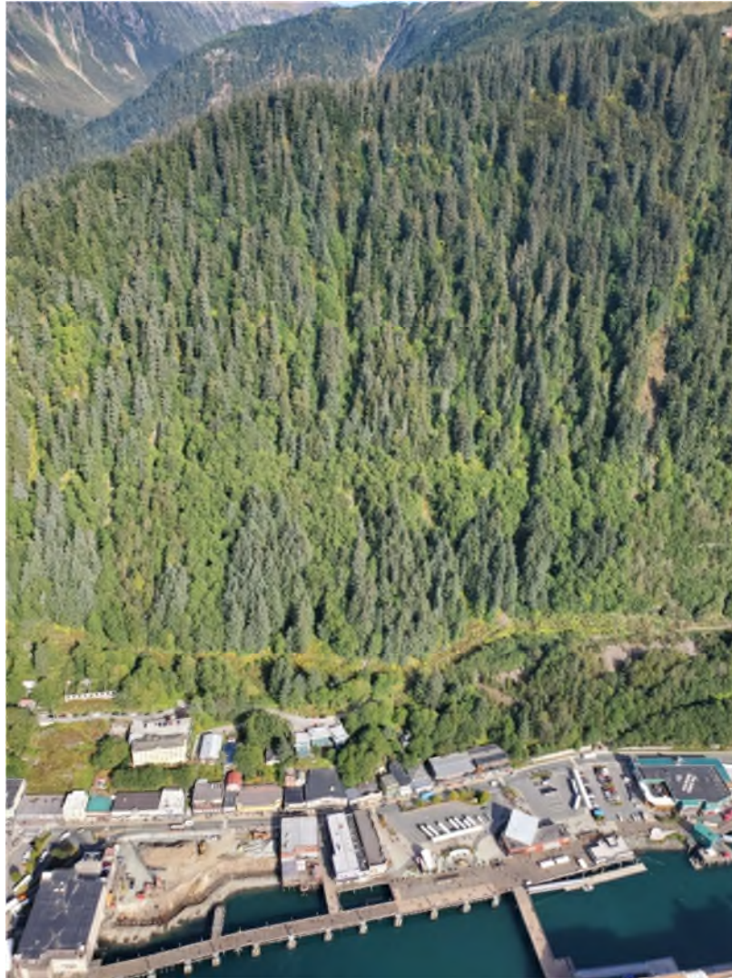
Figure 4a: View of Mt. Roberts from the helicopter showing part of the slope mapped in Figure 3. Note the increasing height of slope from left to right (northwest to southeast). The slope is fairly well-treed but is still prone to avalanching. Gullies tend to increase avalanche runouts. See also Figure 4b.
