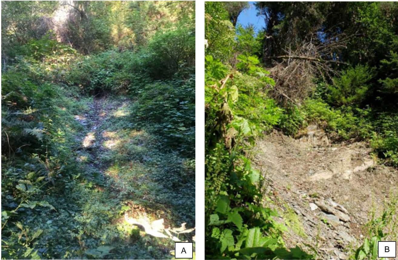
Figure 18: Compares Tetra Tech’s photo from September 10, 2019 (Figure 18A) with residents’ photo from August 1, 2021 (Figure 18B) at the same location. Slope instabilities appear to be ongoing in the historical slide paths located above Nelson Street on a slope with a landslide hazard designation of Severe. See Technical Memo #3 for more information about the slopes around Starr Hill.
