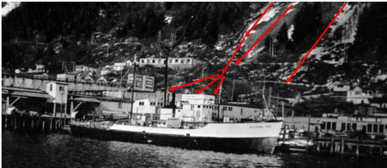
Figure 6: Two apparent debris paths from November 22, 1936, landslide (red arrows, see also Figure 1a, 1b attached). Structure at center-left was the Juneau Cold Storage Company building, later replaced. Debris ran up against the S. Franklin St. side of Juneau Cold Storage, moved the Madsen Building downslope, destroyed several buildings, and killed 15 people. (Photo credit: Alaska State Library – Historical Collections, ASL-P134-312-4 , date uncertain, cropped to fit. ASL 2022d.)
