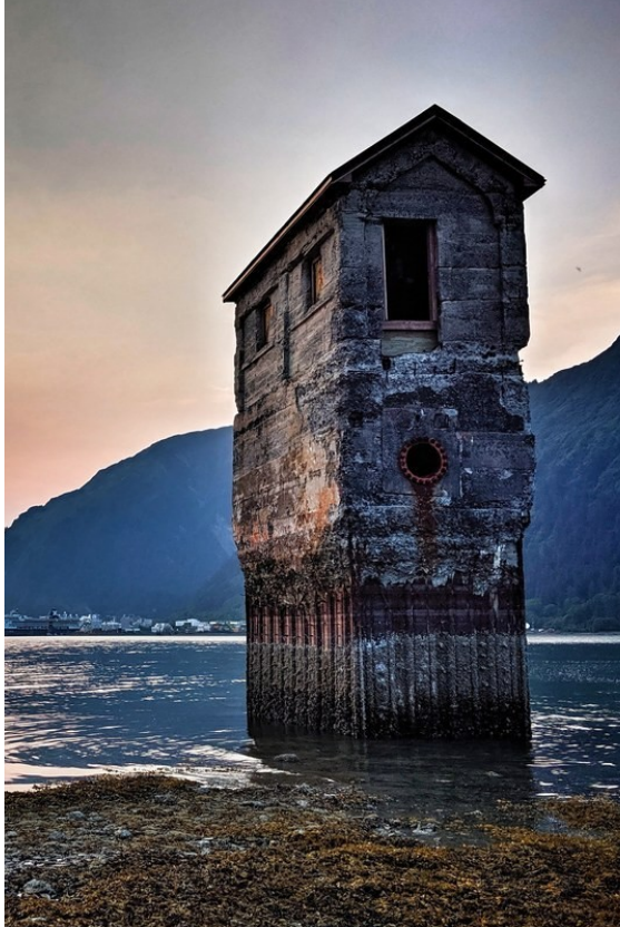
Old Treadwell Pump House. Photo Credit: Patrick McGonegal
