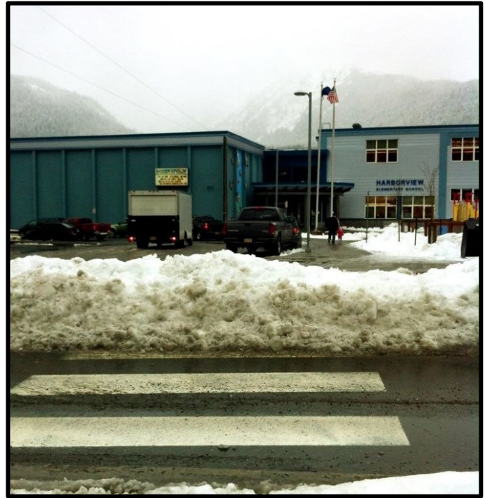
Snow plows leaves a berm in the middle of the main school crosswalk to enter Harborview on Glacier Avenue. Better snow removal practices are needed.
