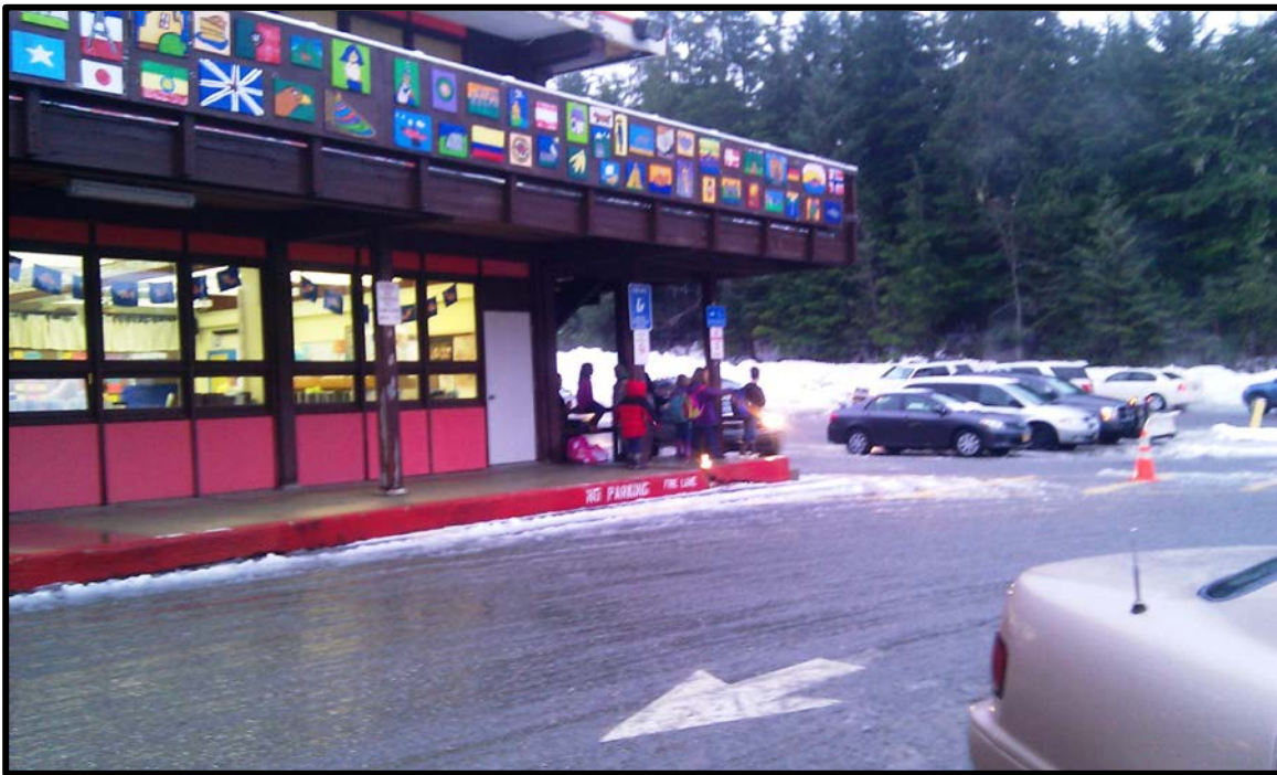
Entrance to Auke Bay Elementary School
