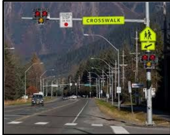
Pedestrian-activated crossing signal on Mendenhall Loop Road by Floyd Dryden Middle School
