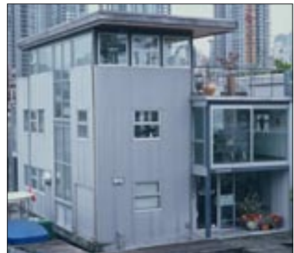
Industrial metal panels combined with large glass plate. (Vancouver, BC)
