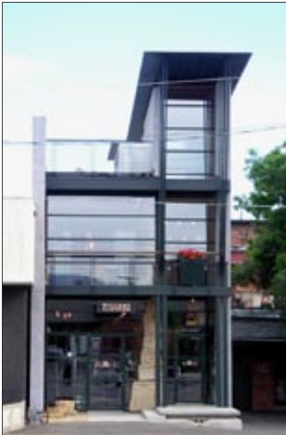
Express facade components in ways that help to establish scale. (Bozeman, MT)
