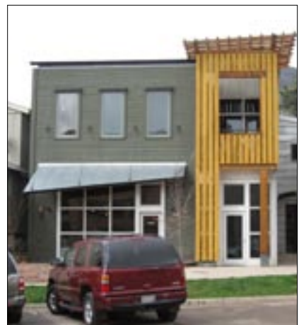
Wood and masonry combined with a contemporary metal canopy. (Basalt, CO)
