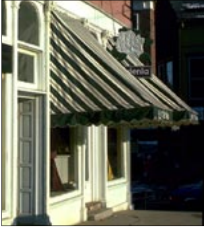
Operable awnings shown here are not permitted.
