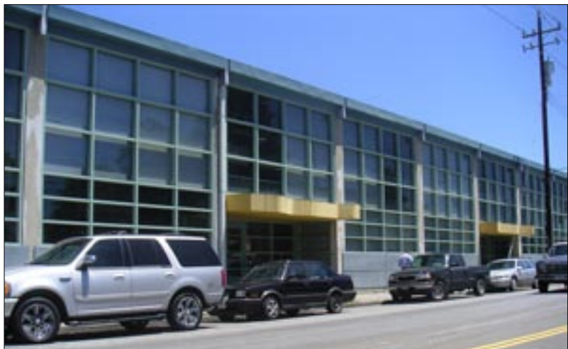
A contemporary interpretation of industrial sash for a commercial building. (Oakland, CA)
