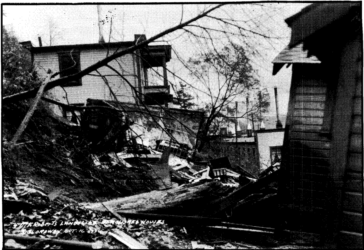
Figure 4. This debris avalanche on Oct. 16, 1936 destroyed buildings between Gastineau Ave. and S. Franklin St. by crushing and relocation. Source: Alaska Historical Library, Early Prints of Alaska Collection.
