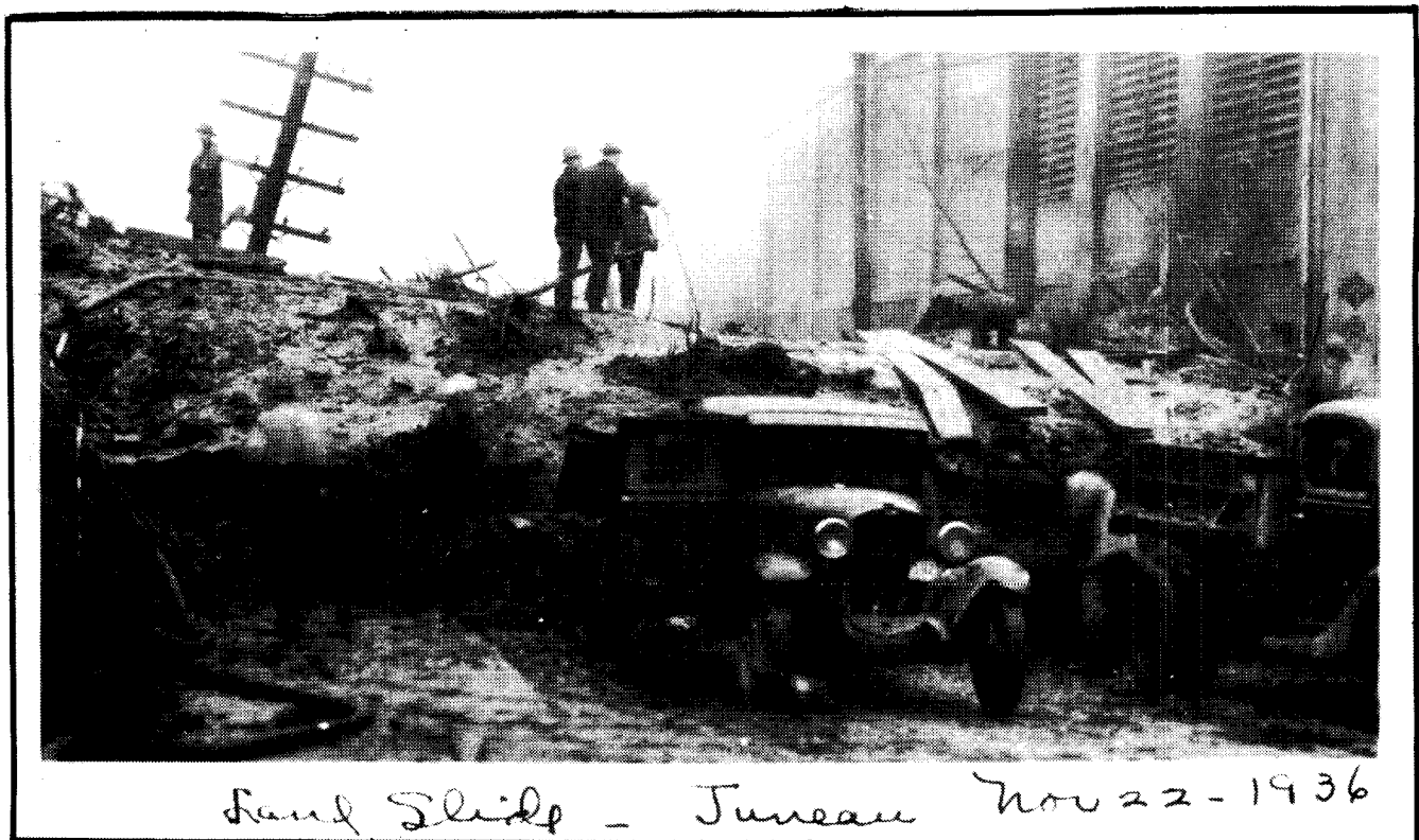
Figure 2. Debris avalanches such as this one on S. Franklin St. (Nov. 22, 1936) exert large thrust pressures against fixed objects while moving and significant depositional forces after movement stops. Flows can be several feet thick and carry rocks and large trees. Source: Alaska Historical Library, Early Prints of Alaska Collection.
