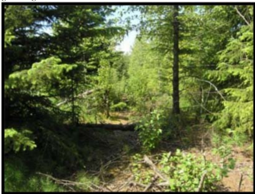
Figure 46 - The dike between sewage #2 and #3.
