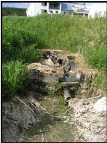
Figure 34 - Outfall for the casa #2 settling pond.
