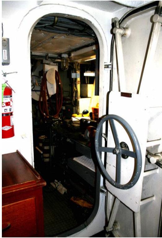
Access to engine room from forecabin looking aft, Sitka Ranger , Sitka, Alaska
