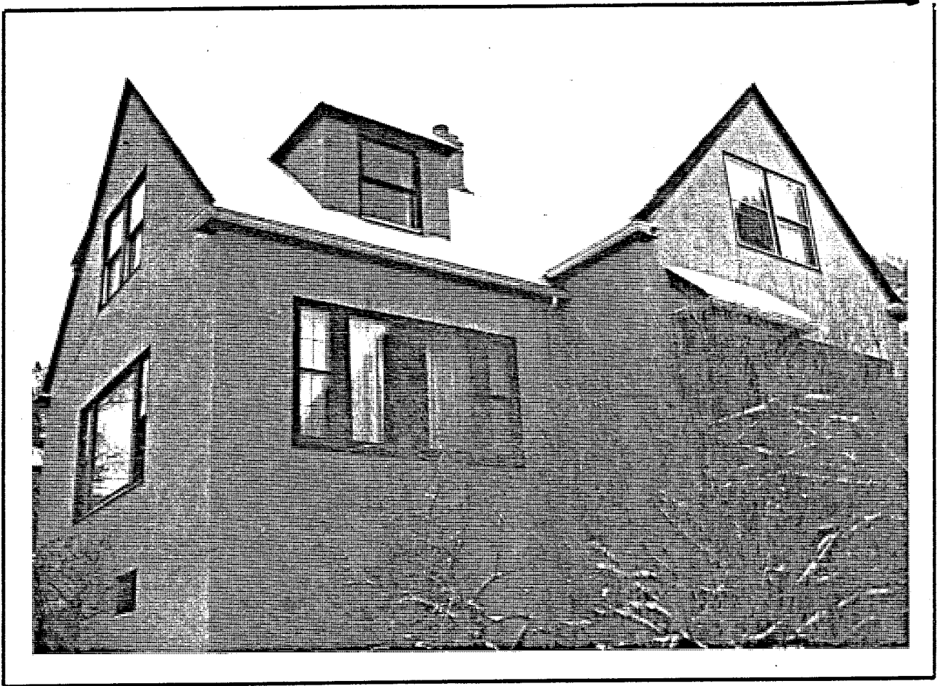
South (Front) and West Facades.
