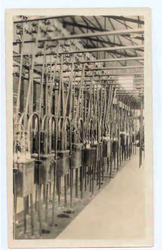
Central Power Plant
