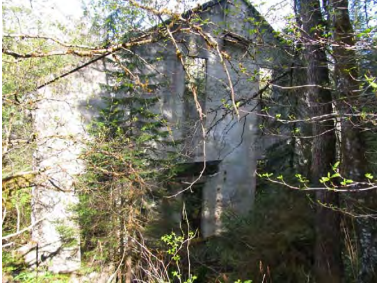
Hoist House, May 2010 Photo courtesy of Wayne Jensen
