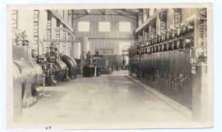
Central Power Plant
