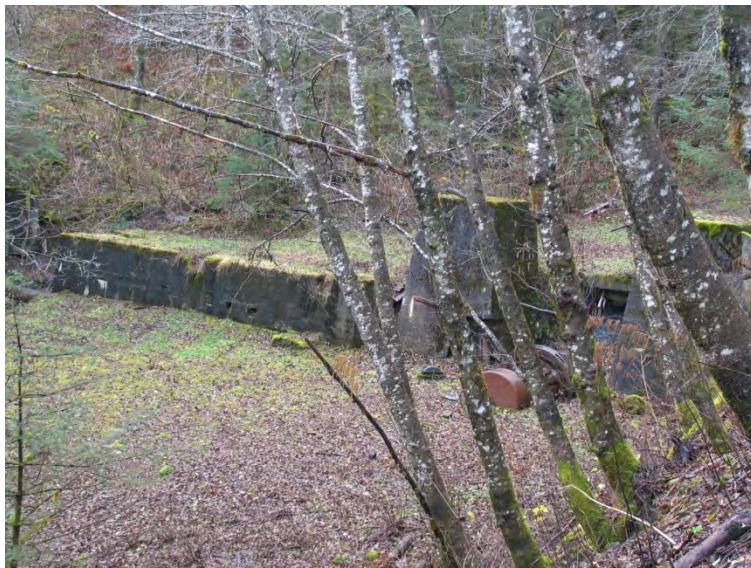
Concrete foundation and electrical generation equipment from 240 Power House, November 2009; photo courtesy of Wayne Jensen.
