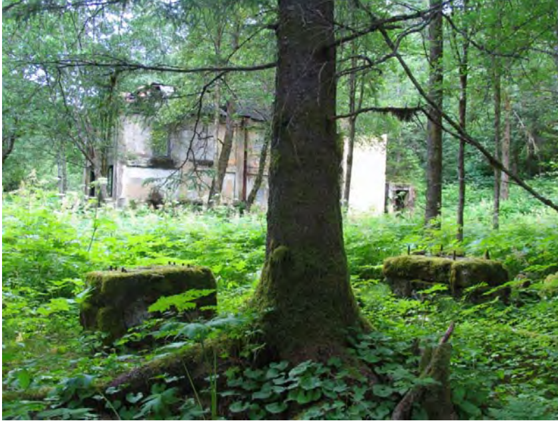
Concrete Foundations in foreground possibly from butcher shop at north side of store. New Office Building in the background.
