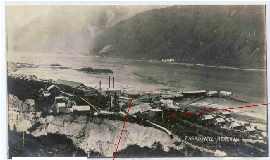
Crude Oil Tank
