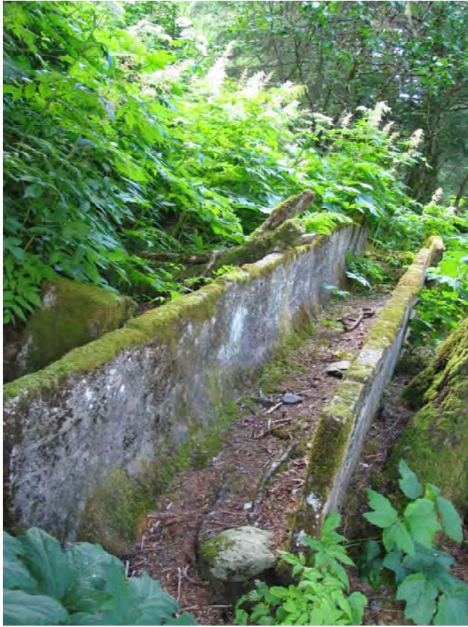
Tailings or wastewater flume from 240 Mill near Treadwell Club Photo by Wayne Jensen
