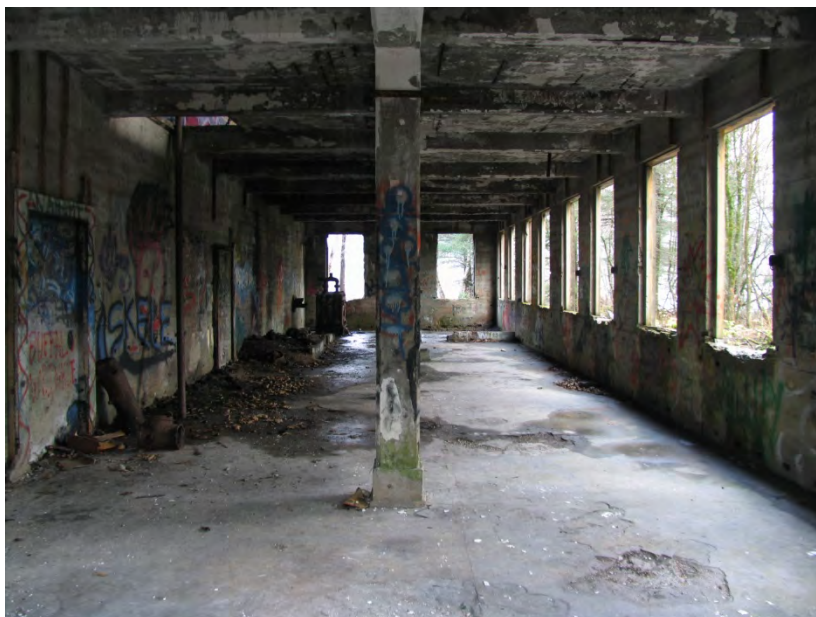
Office building October 2009, Photo courtesy of Wayne Jensen
