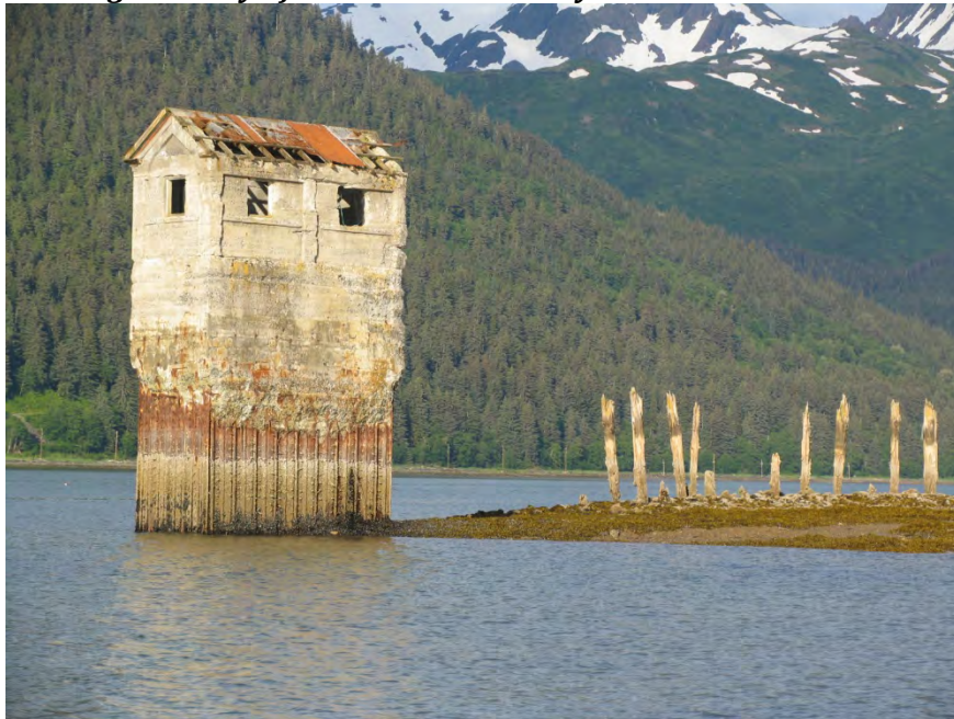
Central Pumping House, June 2010 Photo courtesy of Wayne Jensen
