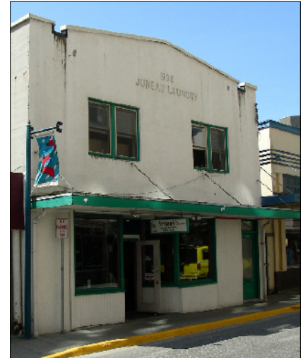
The first step in planning a preservation project is to identify and maintain significant features and materials.
