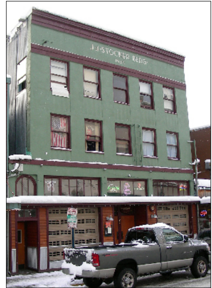
The J. J. Stocker Building (241 Front Street) retains some of its character-defining features, especially from the transom up. This building qualifies as a contributing structure.
