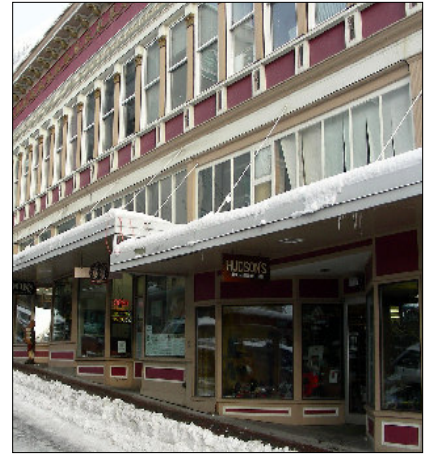
Preserve the historic character of a storefront when it is intact.
