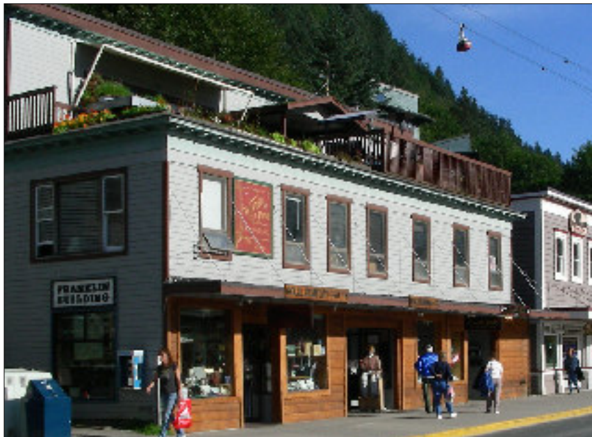
The Madsen's Rooming House (1899, 369 S. Franklin Street) is a contributing structure. The storefront material is a later alteration that detracts. A more appropriate material should match the historic profile and be painted.
