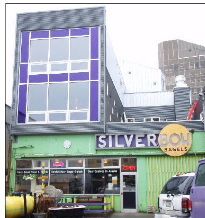
An appropriate rear-facing alley addition.
