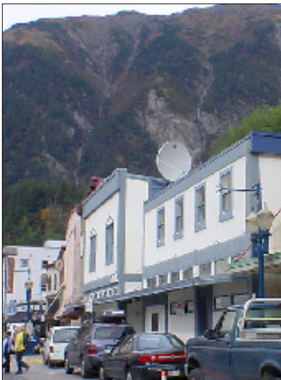
Mechanical equipment such as satellite dishes can detract from the historic character of the downtown when visible from public right-of-ways.
