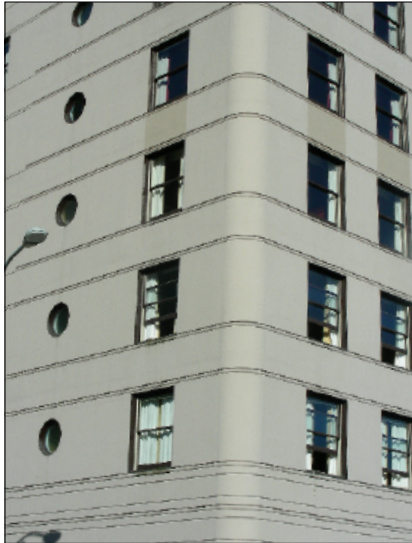
The Baranof Hotel (1932, 105 Franklin Street) has “porthole” windows, rounded corners, and horizontal bands, all characteristic of the Art Moderne style.
