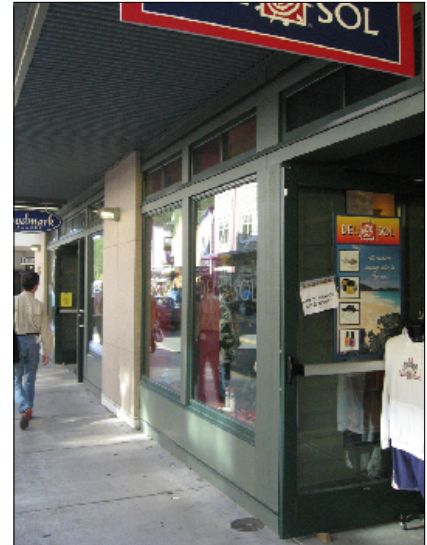
A contemporary interpretation of a storefront including kickplate and canopy, which is appropriate.
