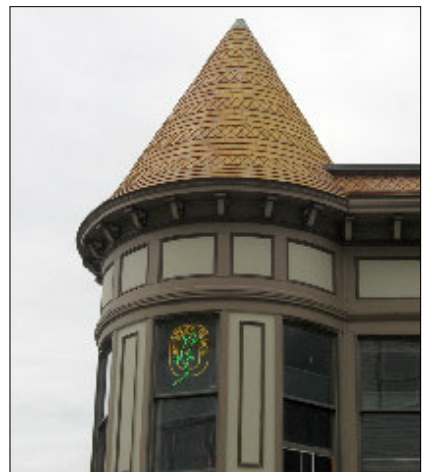
In-kind replacement, as seen on the roof shingles above in 2007, is an option.
