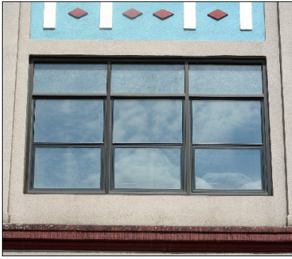
The appearance of window components should match those of the original in dimension, profile and finish.
