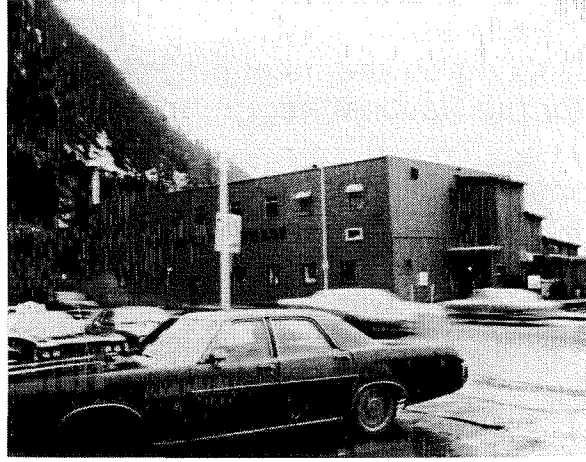
Northwest elevation of Merchant's Wharf building, 1976. Courtesy of CBJ Assessor.
