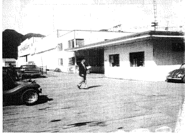
Southwest elevation of Merchant's Wharf building, 1976. Courtesy of CBJ Assessor.
