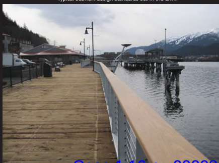
The south end of the completed seawalk. Just outside the rail sits a water sculpture.
