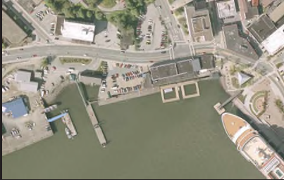
An aerial view shows the existing conditions through this projects extent.
