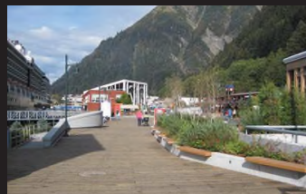
The north extent of this completed section of seawalk.
