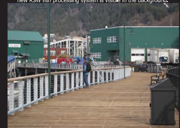
The completed seawalk approaching the Taku Fisheries building from the south.
