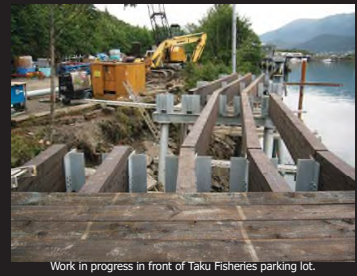
Work in progress in front of Taku Fisheries parking lot.
