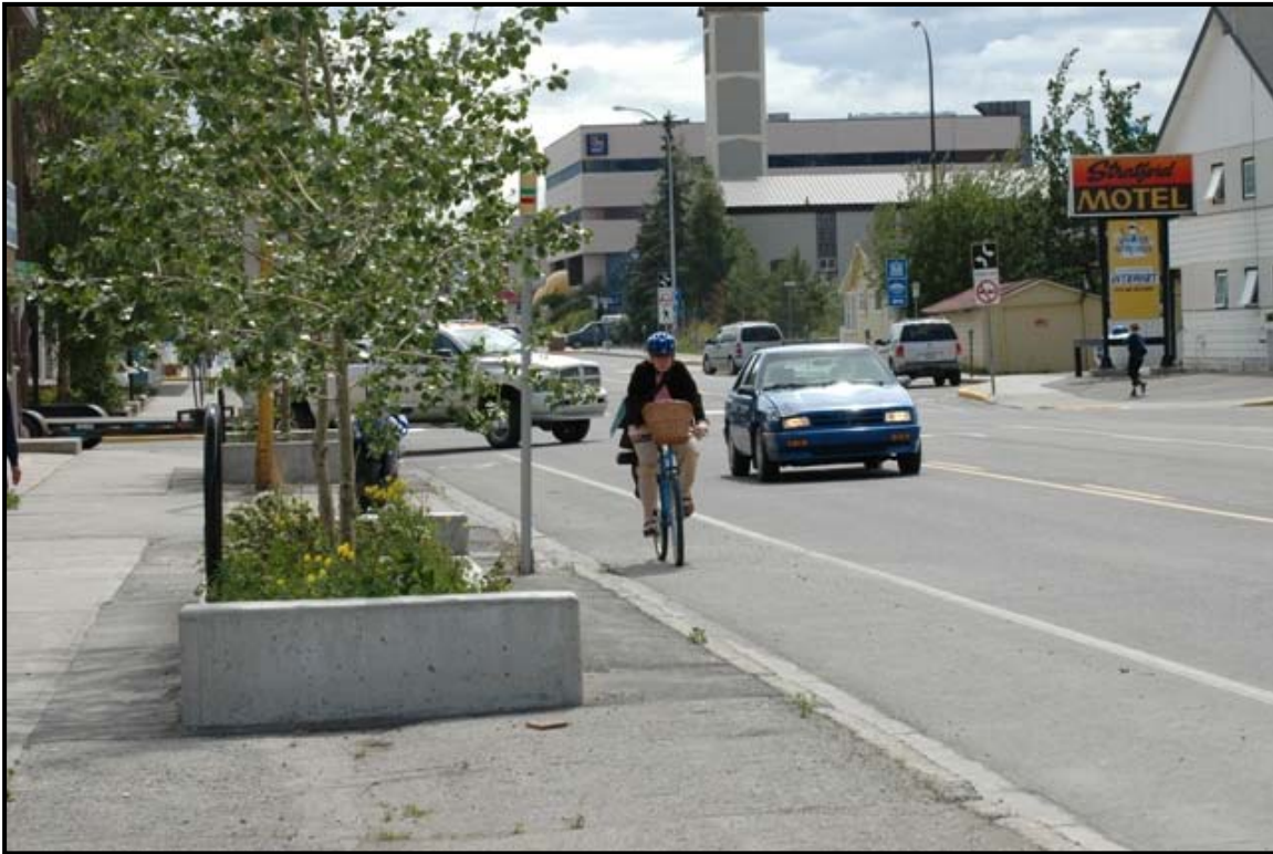
Road Diet - This arterial in Whitehorse Yukon was put on a "road diet". This former four-lane road was modified to implement a "complete street." It has two driving lanes, a center turning lane, bike lanes, curb extensions and a vegetated buffer. (Source: City of Whitehorse)
