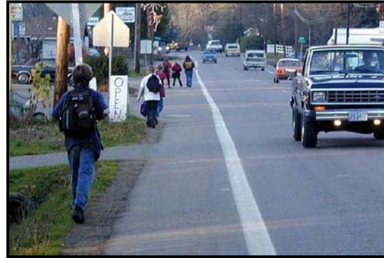
No Sidewalks on a School Route
