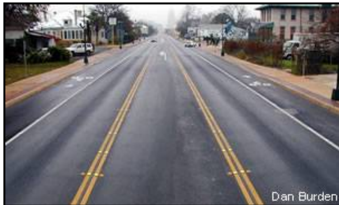
Road Diet (Source: www.saferoutesinfo.org )
