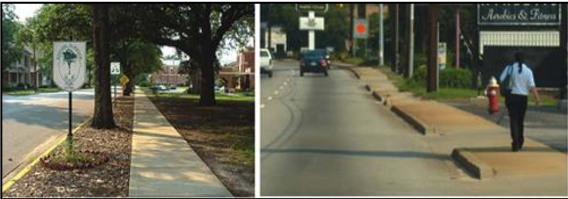
Median and Parkway Landscaping – Photo to the right shows a poorly designed sidewalk and the photo on the left show a well designed sidewalk with buffer (Source: Federal Highway Administration)
