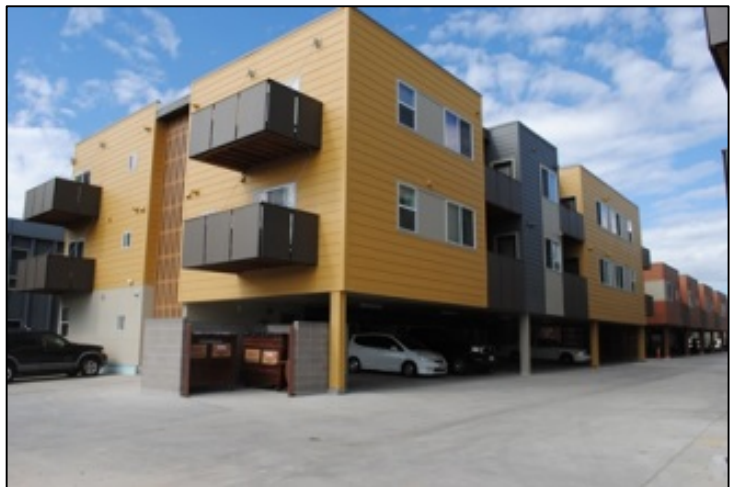
Lumine and Ledges, an affordable apartment project in Boulder, was paid for through cash in lieu payments to the inclusionary housing program, as well as federal Low Income Housing Tax Credits.
