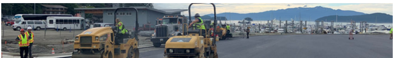
Dawson Construction working on paving for Statter Harbor Phase IIID
