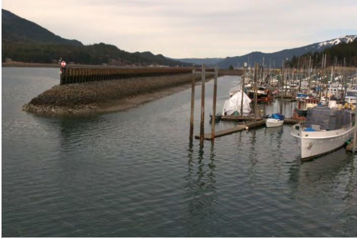
Figure 3: Detached breakwater protecting west side of Aurora Harbor along Gastineau Channel
